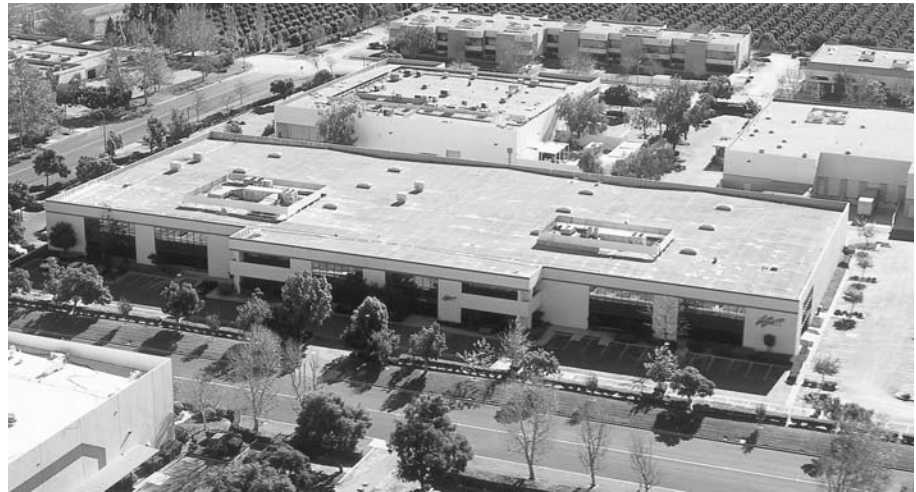
Wilwood Engineering's corporate headquarters.
